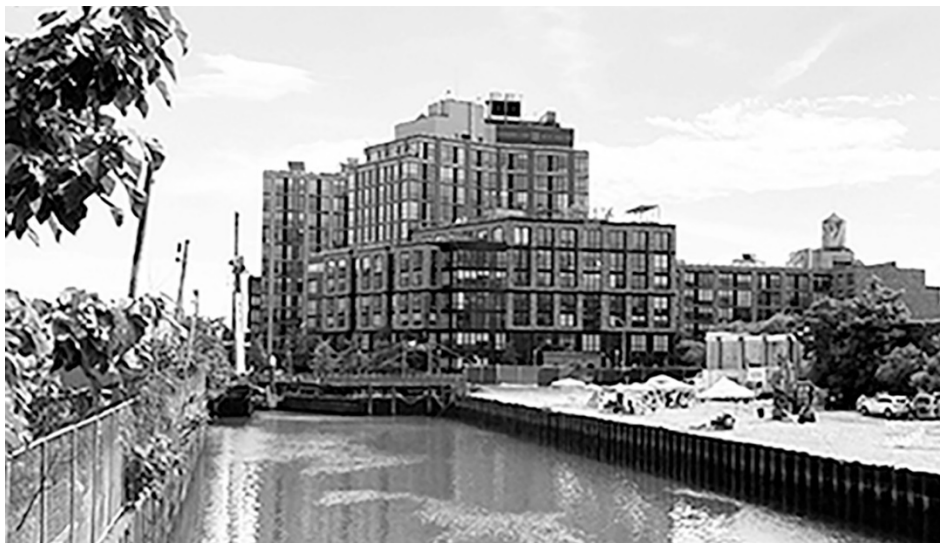
Figure 3. The Gowanus Canal beside the 365 Bond luxury apartment highrise, developed by the Lightstone Group, along with cranes of the Superfund cleanup. Photograph by CM Riley-Duffy.
