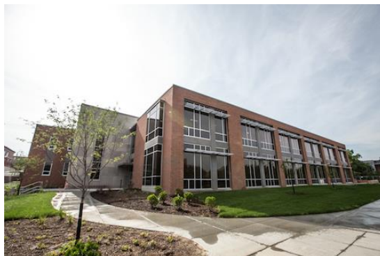
View of Bailey Hall from the east.
