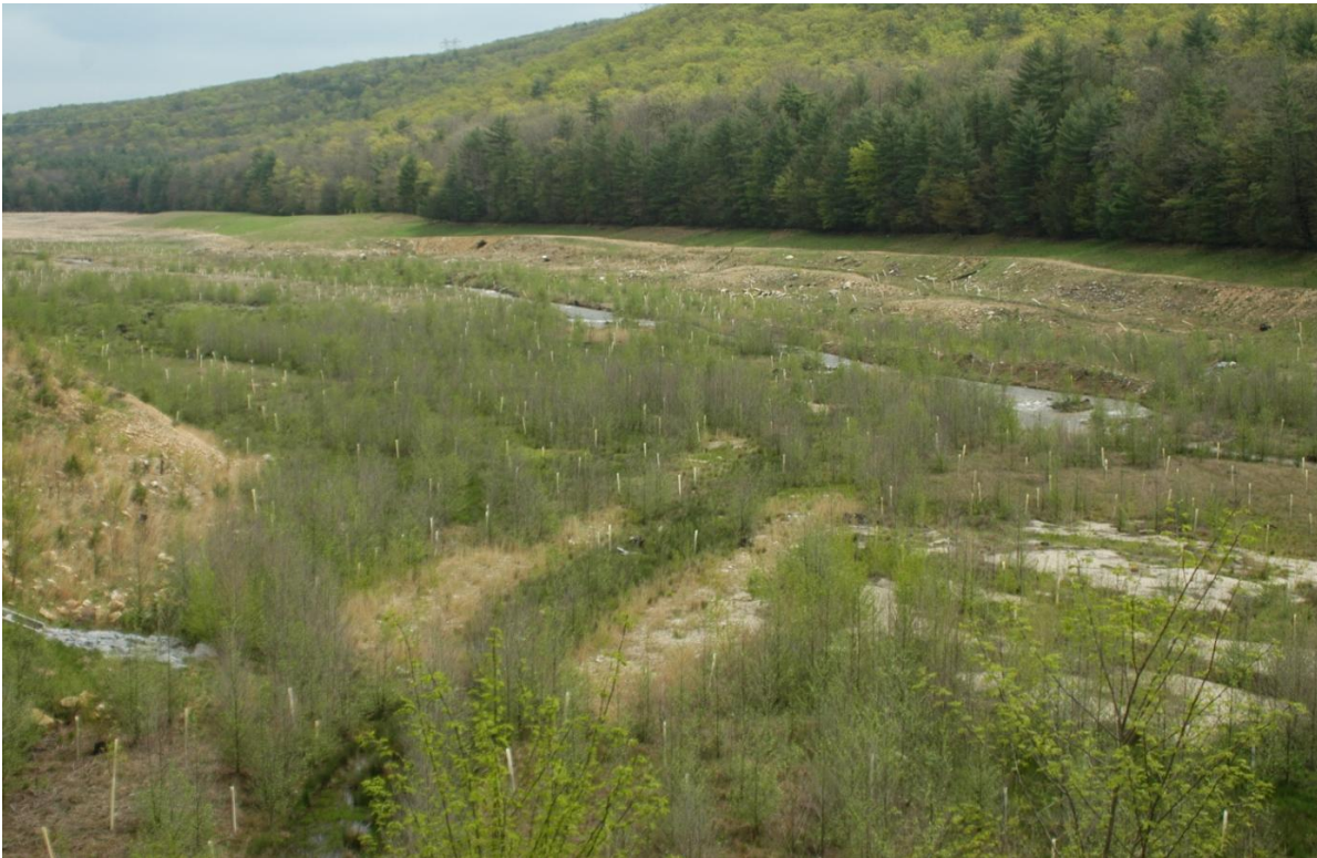
Figure 2. Photograph of the valley formerly covered by the Chambersburg Reservoir. Image is taken from atop the former Birch Run Dam looking east. Conococheague Creek can be seen on the far side of the valley travelling towards the viewer. The temporary channel that led to the dam outlet works can be seen as a green path leading to the foot of the dam. Large deposits of sand are to the right of the abandoned channel (Author's image, 7 May 2009).
