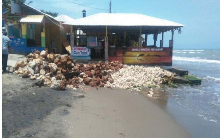
Figure 6. Artificial sea wall at business establishment.
