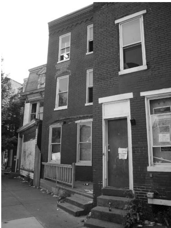
Figure 8. A group of abandoned and vandalized buildings in South Allison Hill.
