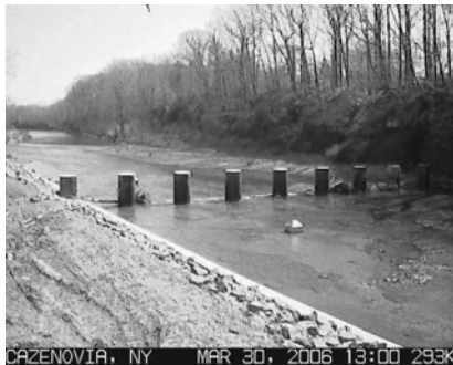
Figure 1. Cazenovia Creek ice-control structure.
